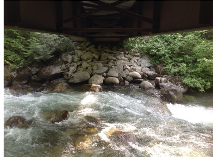
Left Bank Abutment when facing downstream
