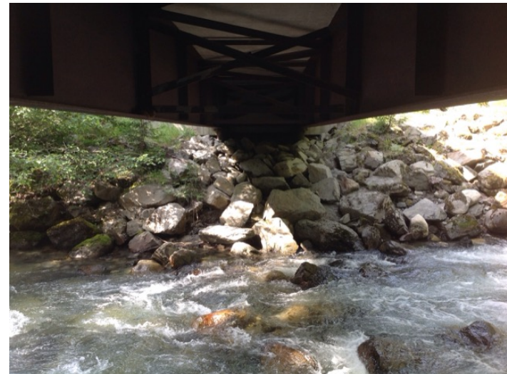
Right Bank Abutment when facing downstream
